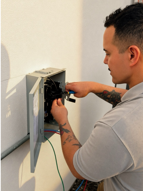
FIELD PHOTO 02 Working at the AC power disconnect.
